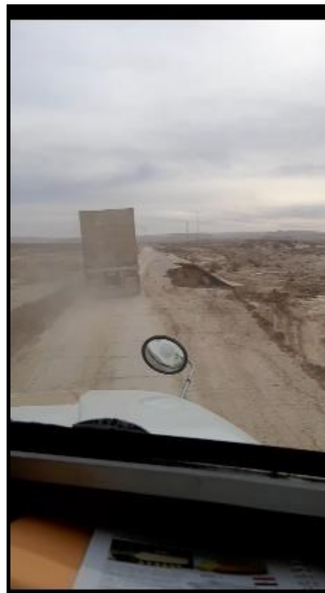
The route from RS2 to RS1 also had damage to the roads due to the storm. This route was also closed for a couple of days until Uruguayan plant operators cleared a section of road that was covered in mud and sand. The engineers did some reconnaissance on this route and it is no longer used by MFO vehicles as it is deemed unsafe due to the road condition. An alternate route is now being used.
