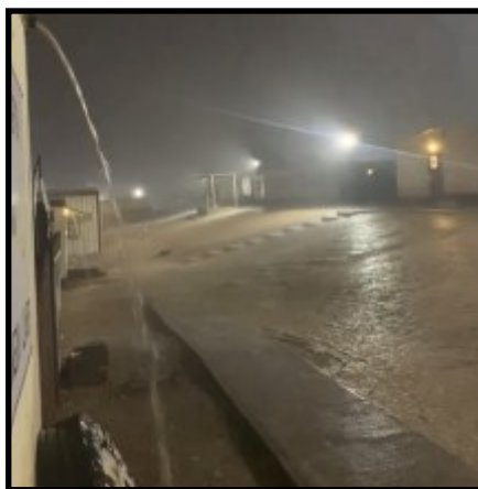
L: The gutters not handling the amount of water coming down.
