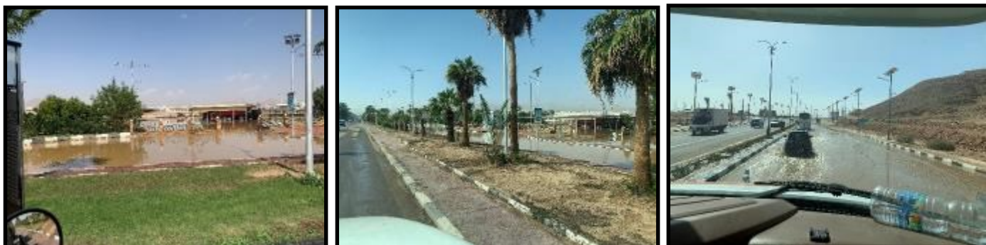
The flooded roads of Sharm El-Sheikh. Sharm does not have any gutters or drains so the water had nowhere to go.
